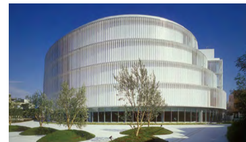
Tokyo Ubiquitous Building
